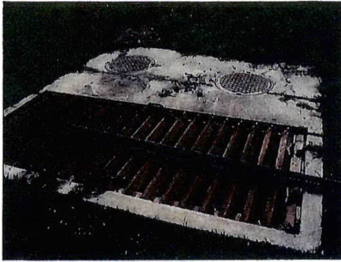
Figure 15: Water and Oil Separator
