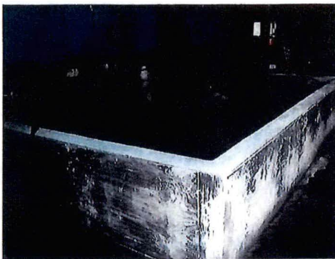
Figure 11: Containment area for the oil containers in the maintenance building
